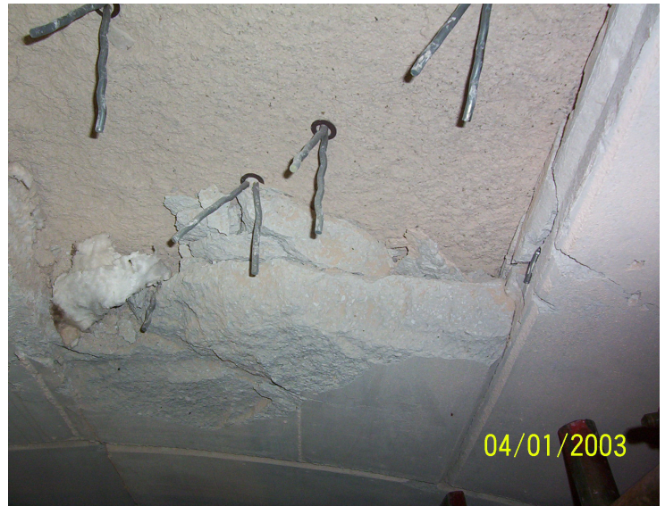
Figure 4 - explosive spall in a gas duct of an iron reduction facility.
