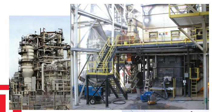
Hotwork provides whole unit heating for: refractory dryout, chemical cleaning, steamblows, turbine operation and component heating of: ash hoppers, burners, ducts, cyclones, curbs, floors, flues, target walls.
