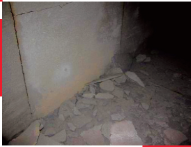
Explosive Spalling
