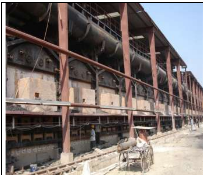
Figure 11: Heatup of a 60 oven heat-recovery coke battery in India in 60 plus days using coal.
