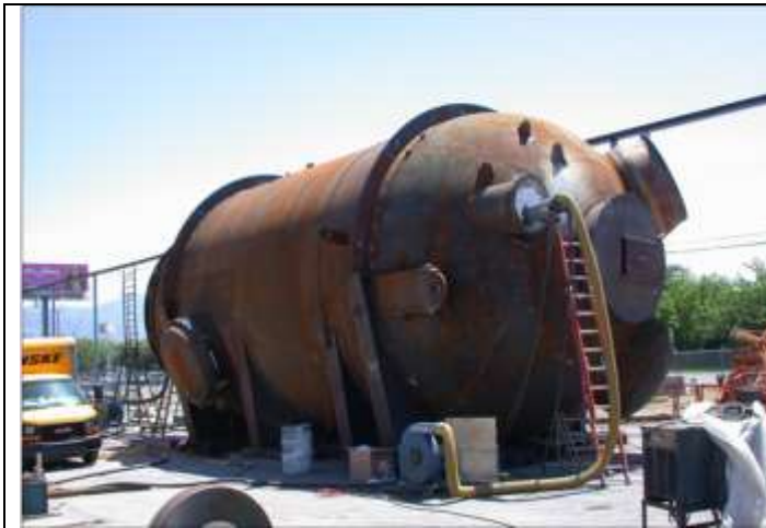
Figure 17: Oil Refinery - 3rd Stage Separator
