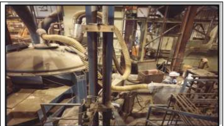
Figure 20: Iron Induction Melting Furnace
