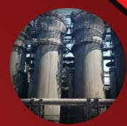
Hotwork patented accelerated heatup of coke ovens in the early 1990s. Today, our 120-hour heating schedule is the industry standard for through-wall repairs. Hotwork has also provided accelerated heating services for non-recovery coke ovens, heating them from ambient to over 2000°F in under
