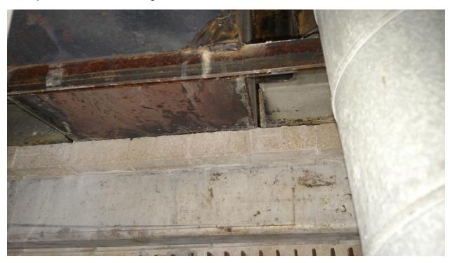
We believed we were setup with the trough at the bottom of the sidewall block but, in fact, the bottom of the sidewall block was at the bottom of that course of brick.
