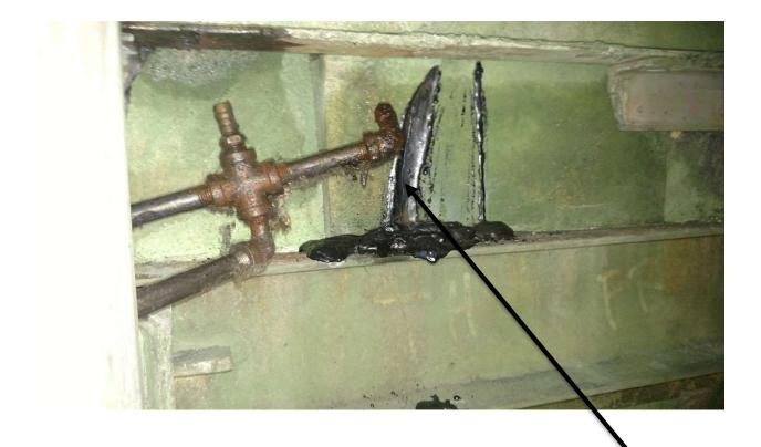
Metal that had leaked out and under the Hotwork trough, through a void that was created in the refractory due to OXY lancing. All lancing was aborted after this point. Due to the concern of the void. If glass entered the void, there would be no way of controlling the leak. This is a major safety concern for the Hotwork crew on site as well as the safety of the plant.
