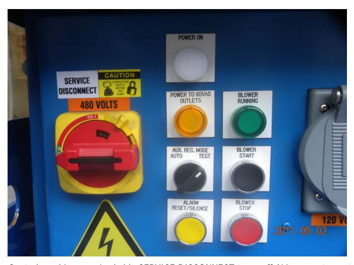
Blower Controls and Lamps. Lockable <u>SERVICE DISCONNECT</u> turns off ALL power to control box.
