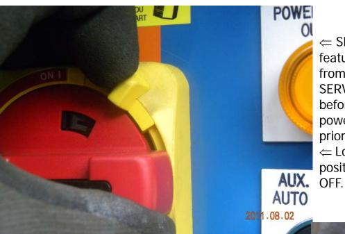
⇐ SERVICE DISCONNECT Has a locking feature that prevents the cabinet door from being opened while energized. SERVICE DISCONNECT must be turned off before attempting to open cabinet. Supply power should be turned off and locked out prior to opening cabinet.
