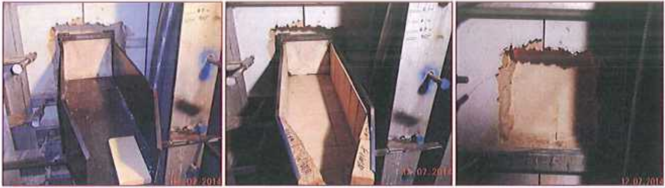
Sidewall insulation removal – cover tile installation into the trough – lining of the trough and installation
