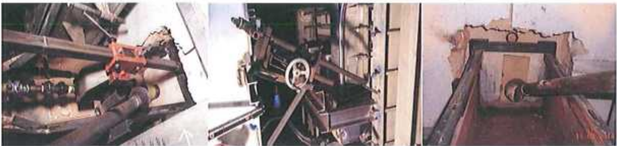
Drilling of the furnace sidewall – set up of the safety ball – hole drilled and a safety brick in front of the hole
